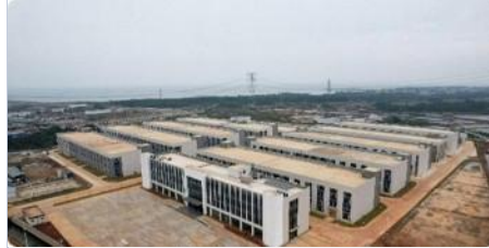
Leizhou, Guangdong Hydrometallurgy Production Base
